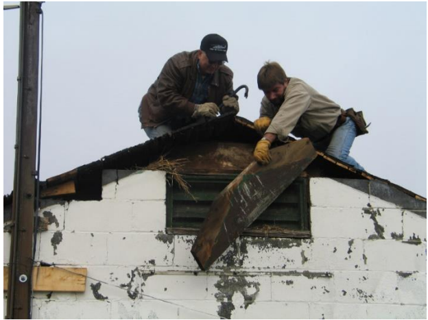
Club members remove old roof and install trusses
